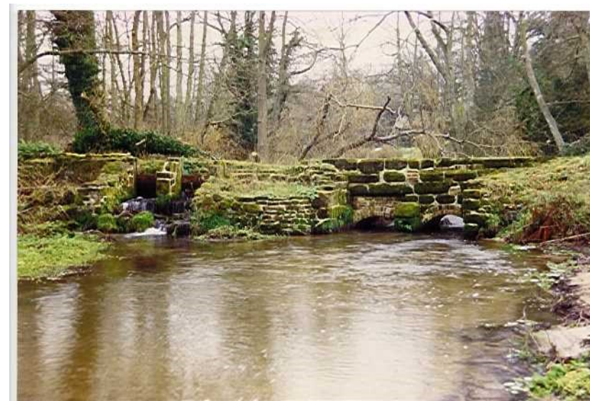
ABOVE A SECOND AQUEDUCT AT BRAMSHOTT COURT IS ALSO A SCHEDULED MONUMENT, AND ...
