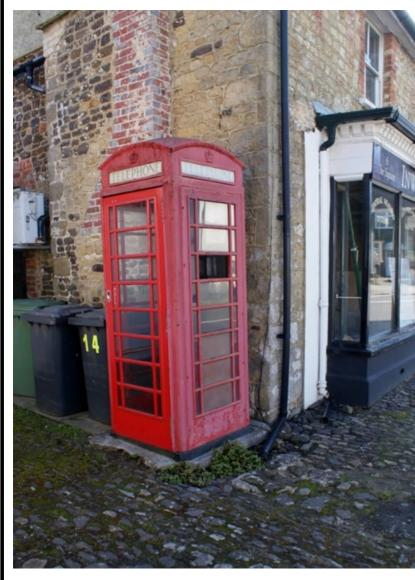
Telephone kiosk. Type K6. Designed 1935 by Sir Giles Gilbert Scott. Made by various contractors. Cast iron. Square kiosk with domed roof. Unperforated George VI crowns to top panels and margin glazing to windows and door.
