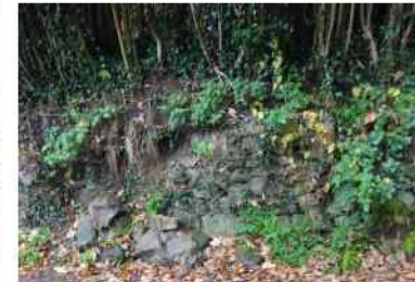
WALLS IN RECTORY LANE DISPLAYING TYPICAL ISSUES — LEFT PROGRESSIVE EROSION AND INSTABILITY DUE TO TREE ROOTS AND WEIGHT; CENTRE PROBABLY DAMAGE BY A LARGE VEHICLE PULLING OVER TOO FAR; RIGHT PROBABLY A MIXTURE OF ADDED OVERBURDEN, RAISED WALL (IN A 'HARD' MORTAR) AND SHRUB GROWTH
