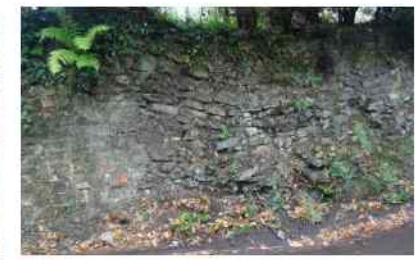
WALLS IN RECTORY LANE DISPLAYING TYPICAL ISSUES — LEFT PROGRESSIVE EROSION AND INSTABILITY DUE TO TREE ROOTS AND WEIGHT; CENTRE PROBABLY DAMAGE BY A LARGE VEHICLE PULLING OVER TOO FAR; RIGHT PROBABLY A MIXTURE OF ADDED OVERBURDEN, RAISED WALL (IN A 'HARD' MORTAR) AND SHRUB GROWTH
